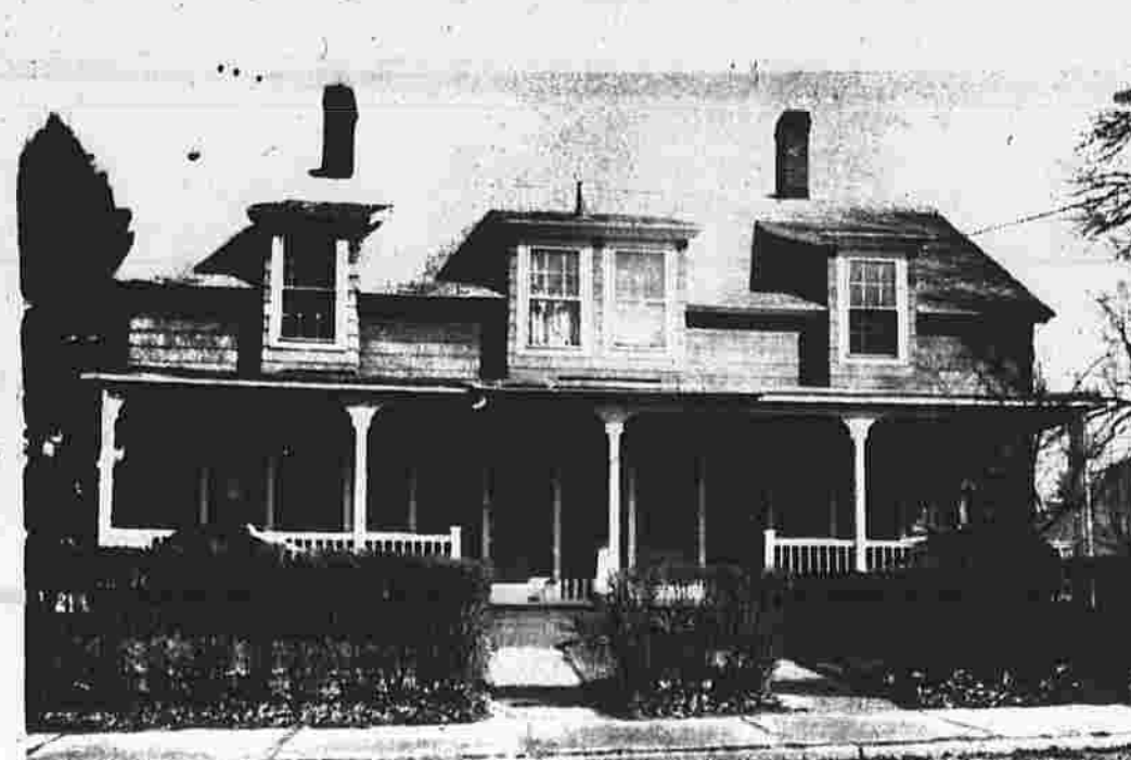
This side-by-side duplex house at 85 and 87 School St. is one of four the Manchester Housing Authority has bought to rehabilitate and rent. Its asbestos siding will get a new coat of paint in the process.
